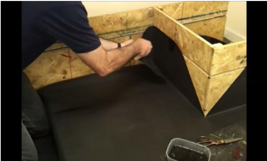
Fig 2: Tying the sheet membrane temporarily out of the way.
