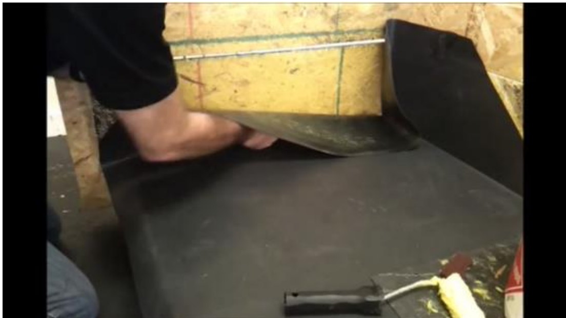
Fig 4: Using the penny roller along the bottom of the upstand wall.
