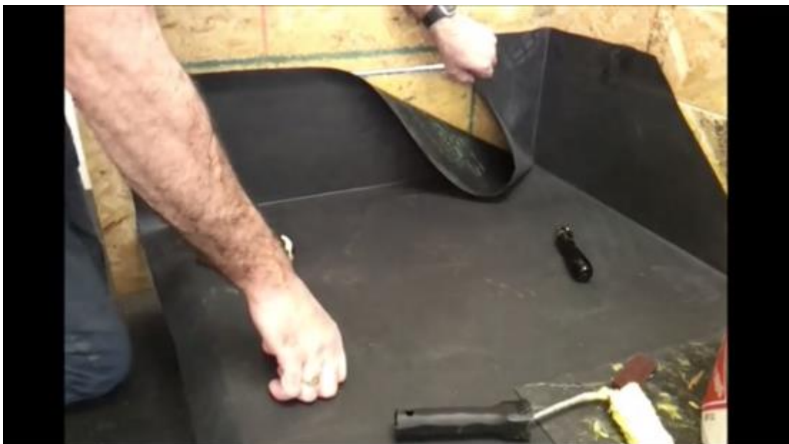
Fig 6: Bringing the membrane over to form the corner.
