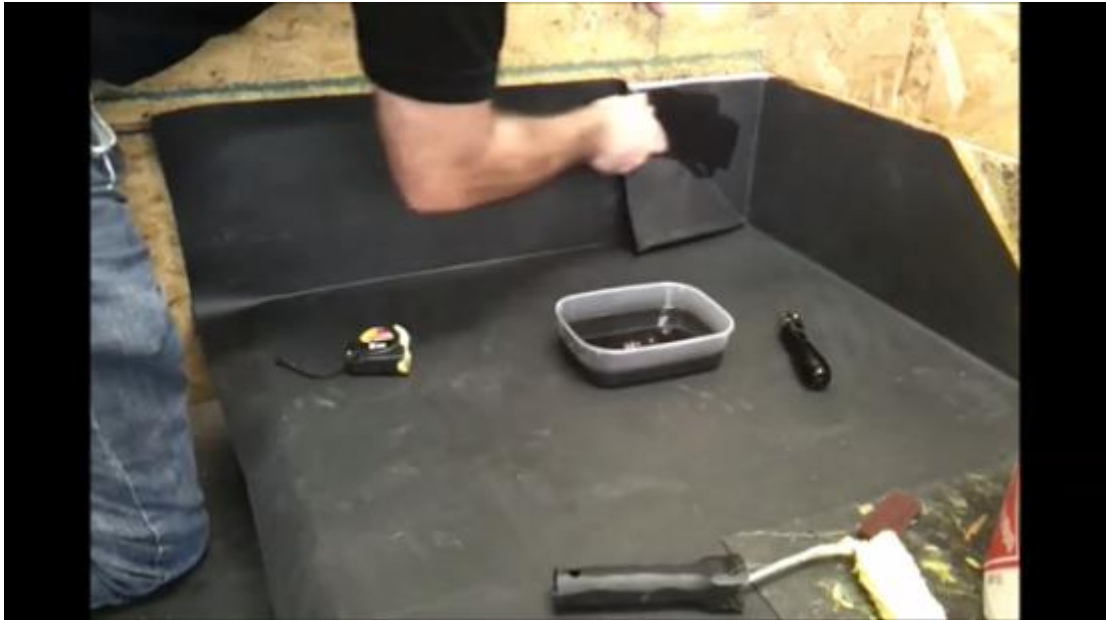
Fig 9: Securing the flap to the back wall with Quickprime Plus.
