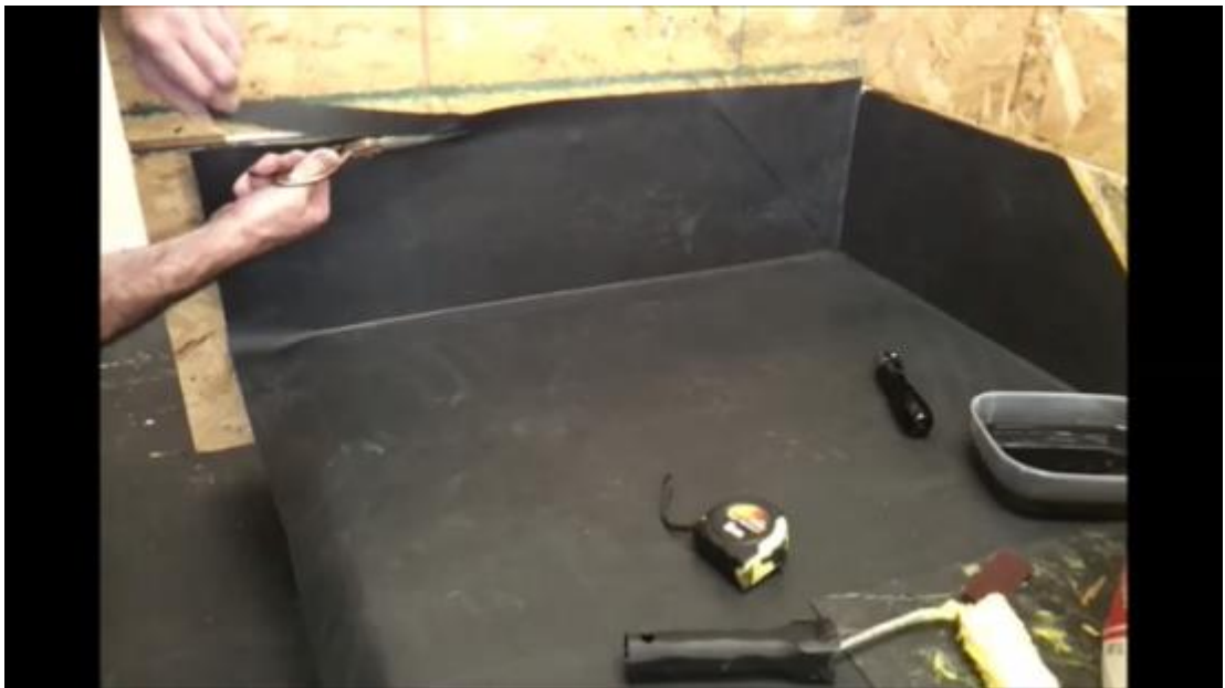
Fig 11: Trimming off the excess membrane.
