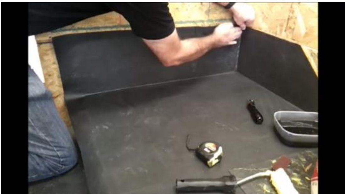
Fig 10: Offering the sheet up to the back wall to secure.
