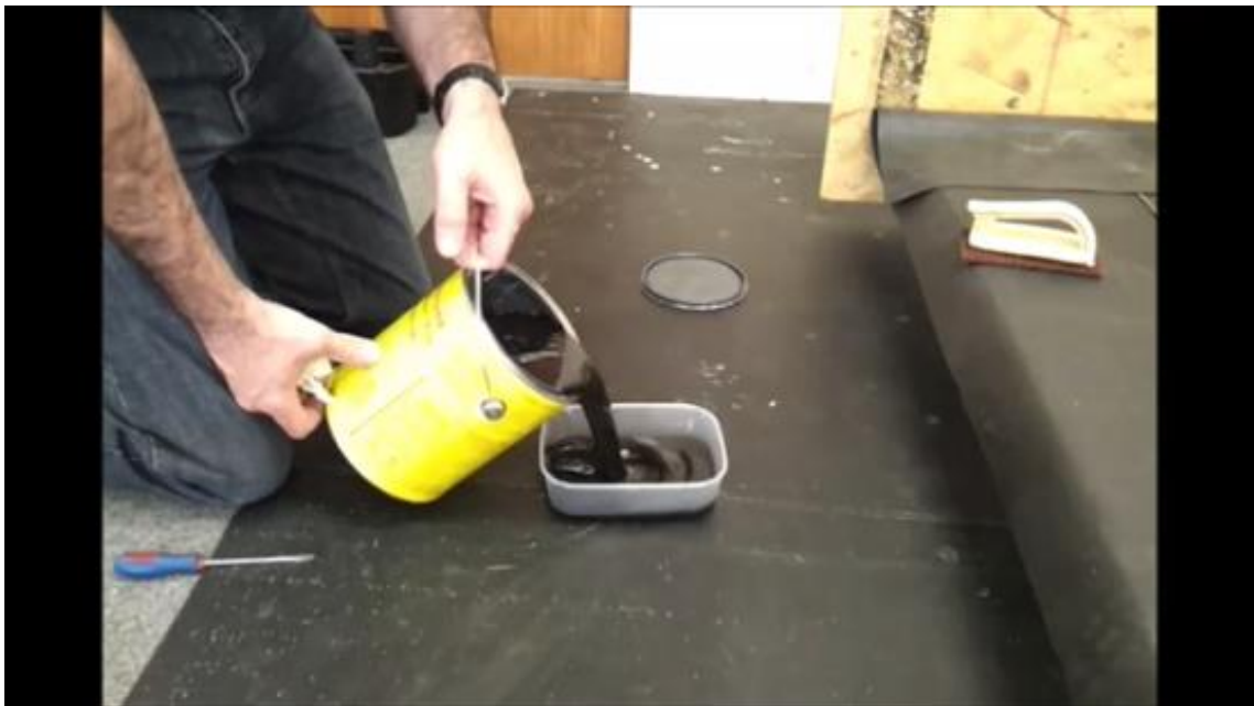
Fig 1: Decanting mixed Quickprime Plus into a small container.
