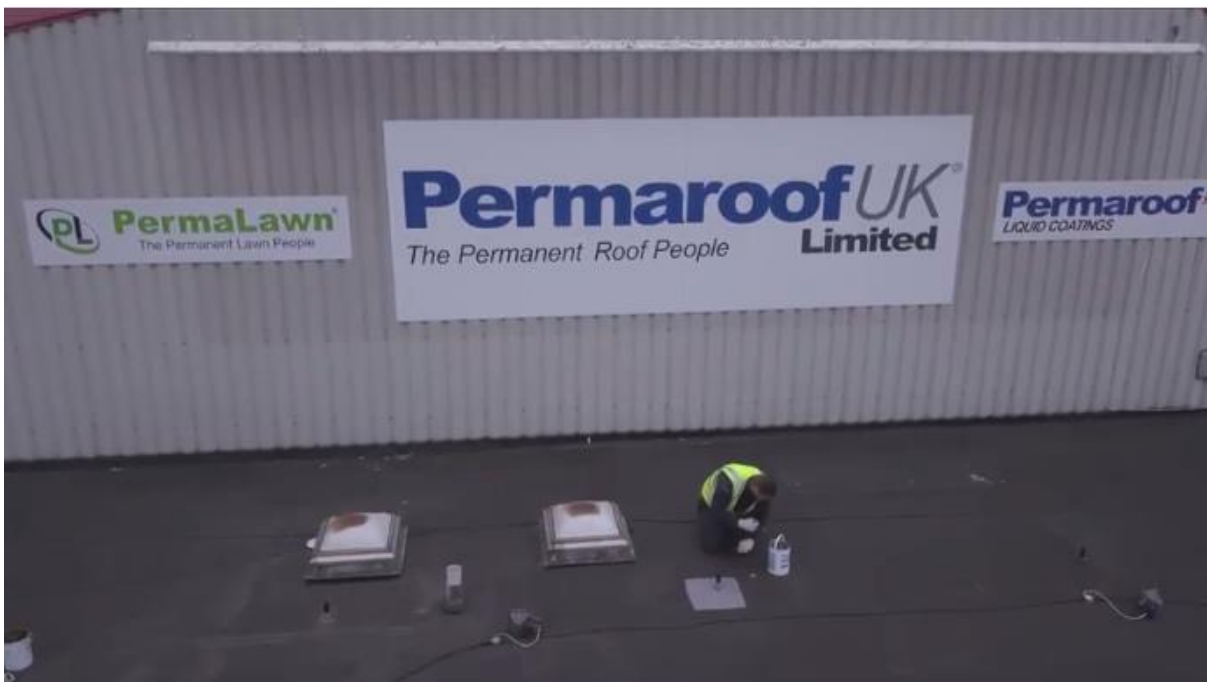
Fig 8 – Viewing the work area from above.
