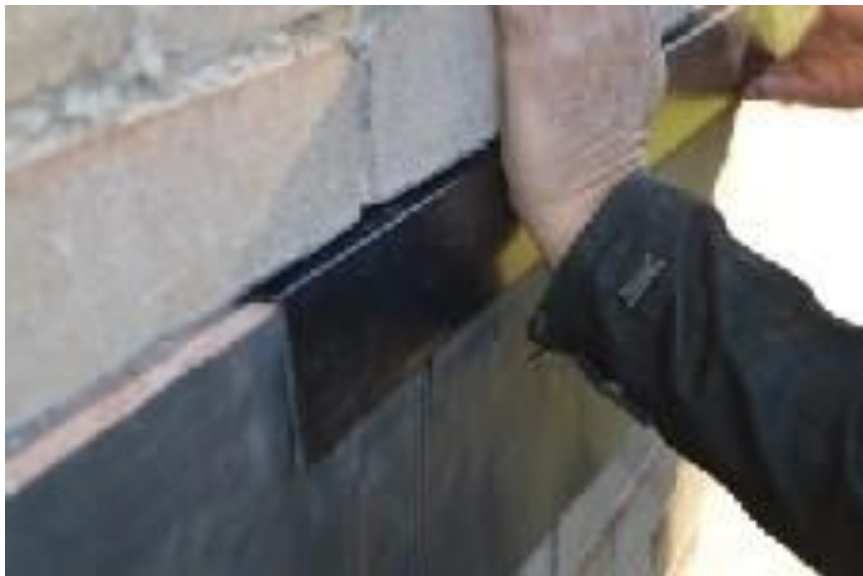
Fig 4: Inserting the Permaroof Wall Flashing.
