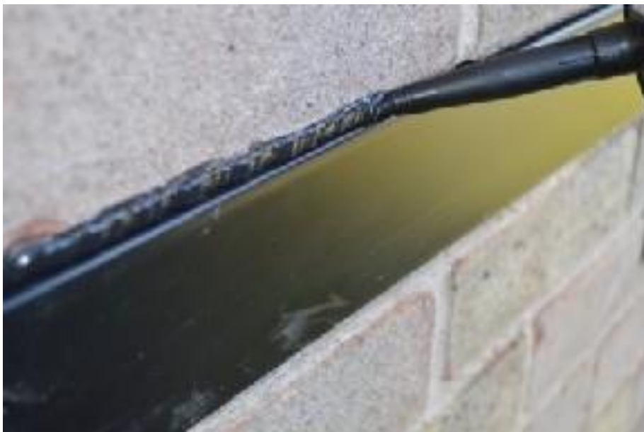
Fig 7: Sealing up the chase with Permaroof Ultrabond.
