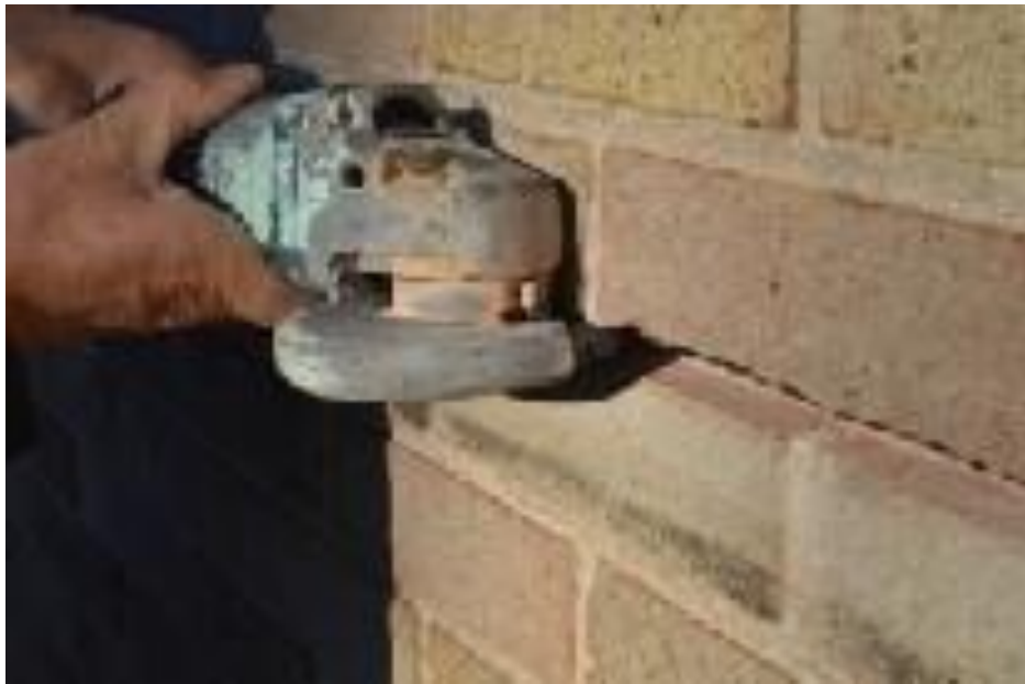
Fig 1: Grinding out the chase.
