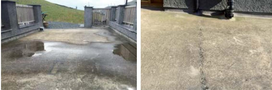
Any small cracks and damaged areas can be repaired with matting embedded in a coat of liquid membrane (**AFTER PRIMING**). Any significant cracks to be filled using any approved polyurethane based mastic (**BEFORE PRIMER IS APPLIED**). **AVOID the use of silicone based mastics.**
