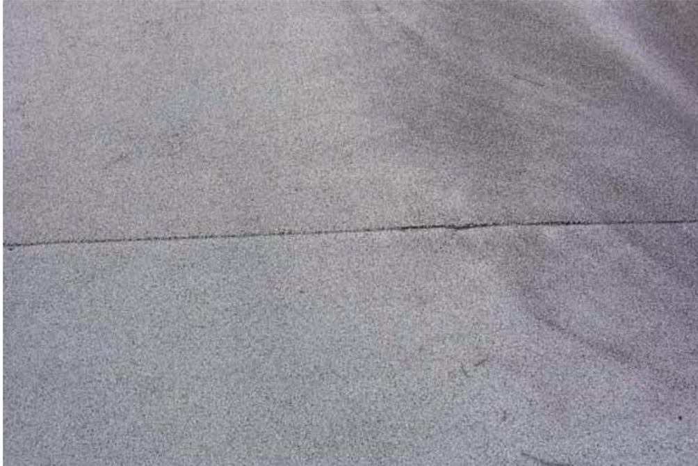
Matting must be used on any joints, cracks or change of materials. Accelerated liquid membrane is applied to the surface, the matting is rolled into the membrane (until liquid membrane is drawn through), then another coat of liquid membrane is applied ensuring the matting is fully embedded.
